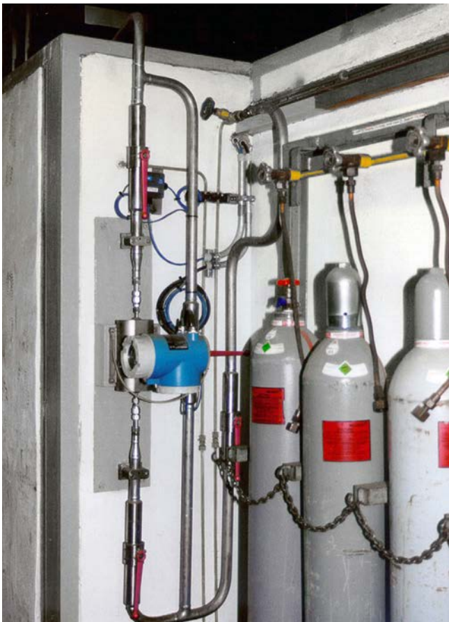
Proline Promass Coriolis flowmeter monitoring the mass flow of hydrogen to control the cooling of the generator
